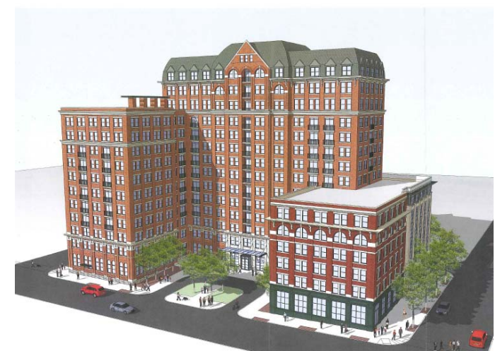
Exterior View from 1 st Street
